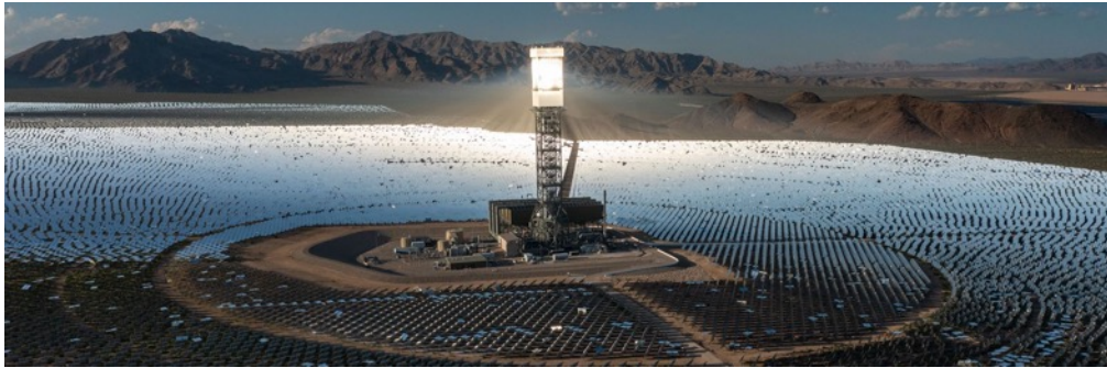
CSP: monolithic, one-off projects, assembled onsite
